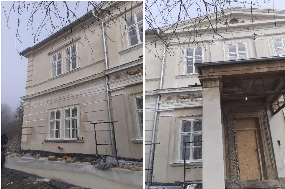
Fig. 2. View of the Dobrovice Parish after the general repair and construction modifications.
